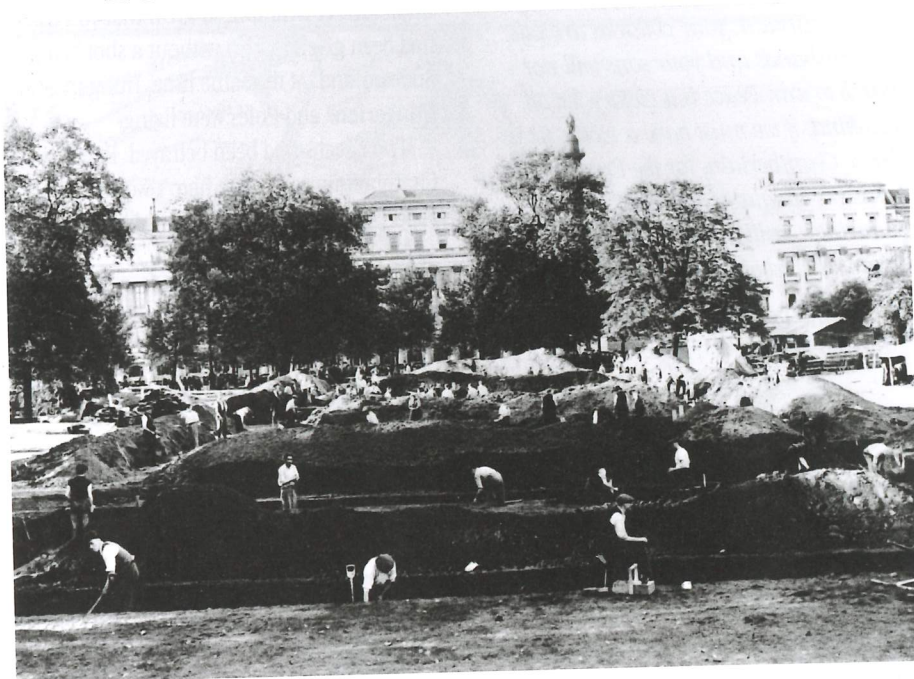
Digging air raid defences in London, September 1938.
